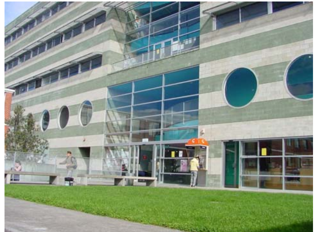
Commerce Building (Hobart Campus)
