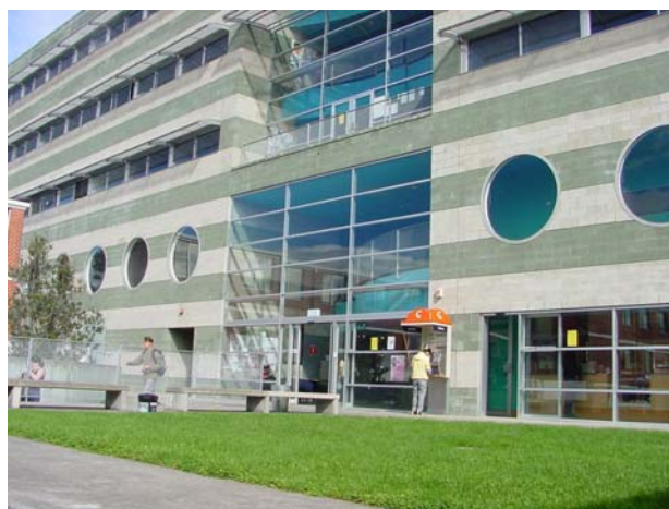
Commerce Building (Hobart Campus)
