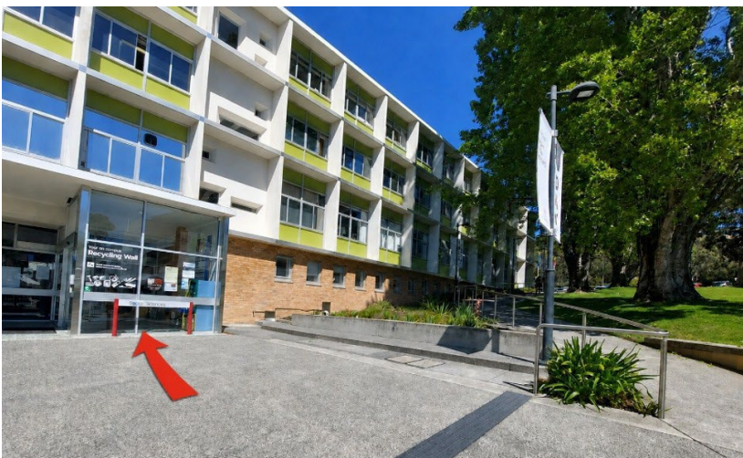
Figure 3 On the right, enter through the glass doors. There will be signage at the front of the building
