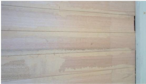
**Slabbing: adhesion and shrinkage**
