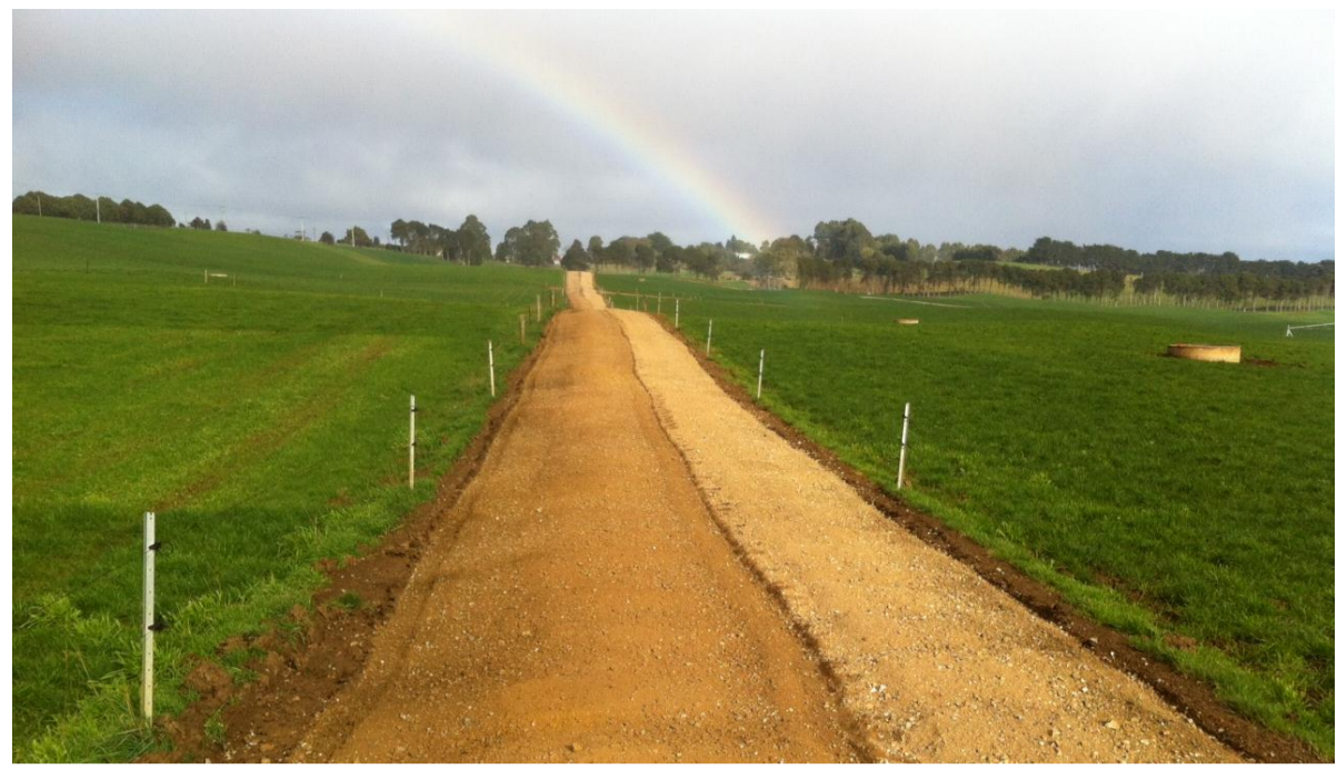
Laneway resurfaced with the stone crusher
