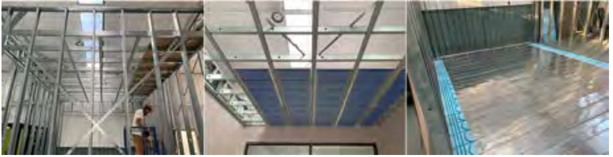
Figure 1: Test cell frame, ceiling, and floor under construction
