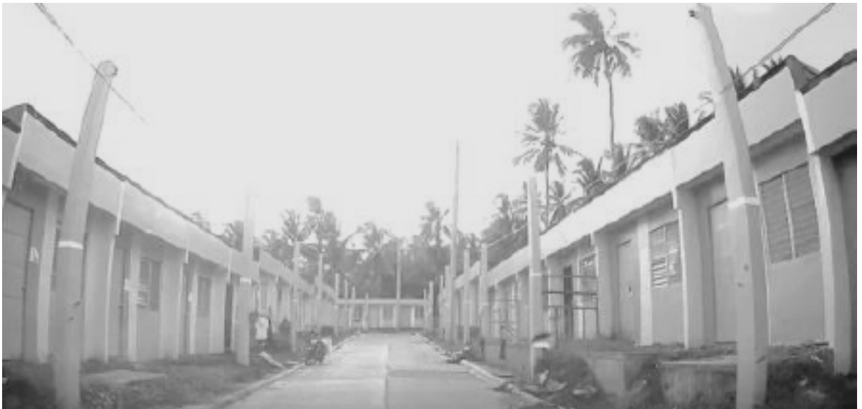
Figure 29: Actual photo of a typical socialized housing unit with an 18 sqm floor area and 35 sqm lot.
