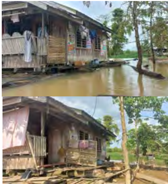
Figure 5: Situation of a hapa floating house during flooding (left) and dry (right) seasons
