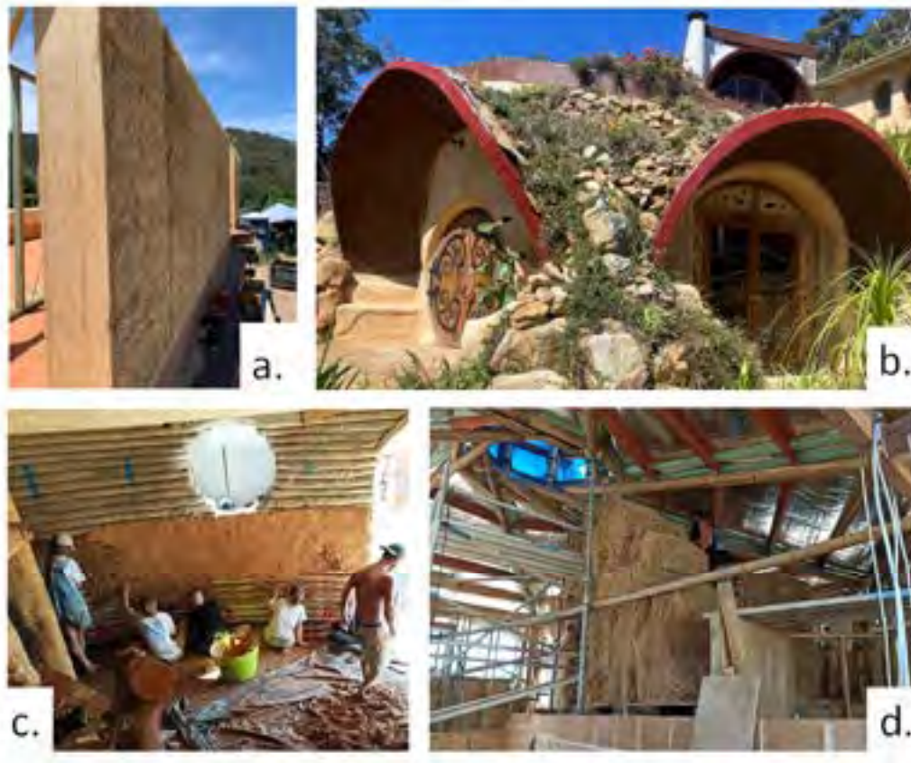
Figure 4 - Building technologies of homes 5 to 7. a. Prefabricated straw panel external wall for home 5 (Source: M. Lloyd); b. Home 6 art studio (Source: L. Scott); c. Home 6 art studio internal wall clay rendering onto super-adobe earth bags (Source: Will Eason); d. Straw baling the internal walls of the octagonal-shaped home 7, with the bamboo reciprocal roof at the top left blue cupola (Source: C. Oosthuizen)
