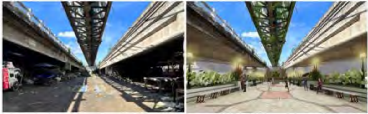
Figure 11: An infrastructural void located under Bangkerohan Bridge proposed as passive and active park
