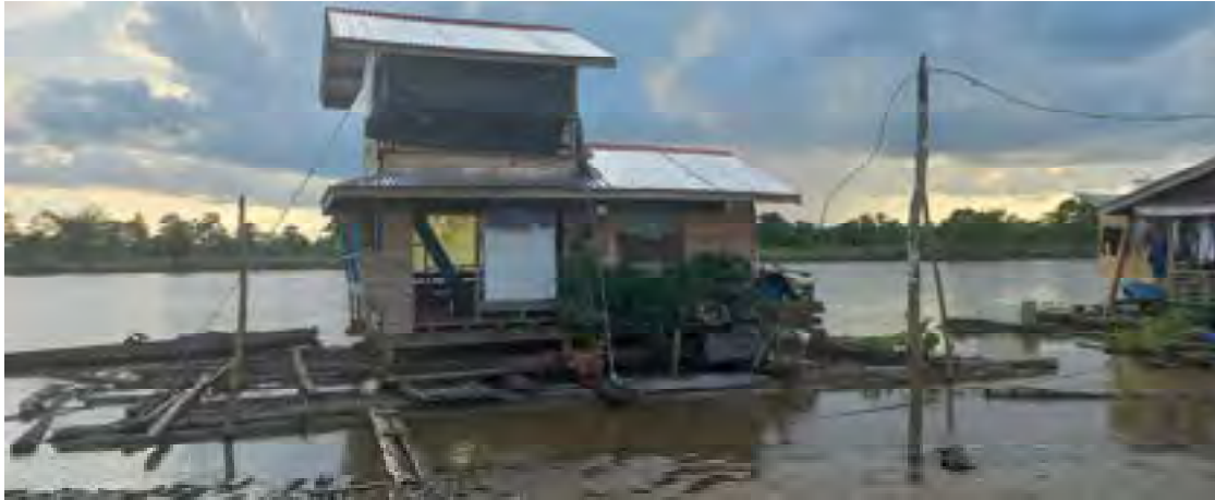
Figure 7: A dos andanas floating house yet to be completed but already occupied by the owners
