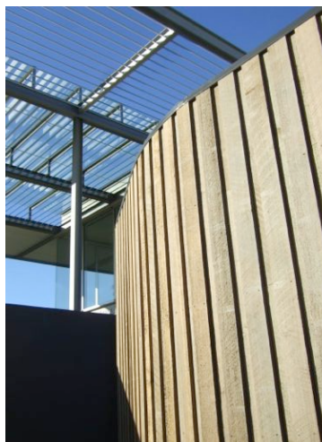
Vertical board cladding
