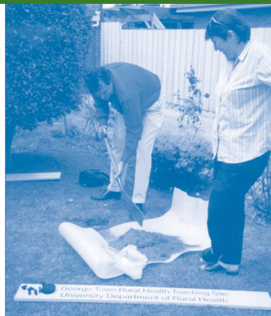
An exercise in multi-skilling - Stuart Auckland digs a hole for the George Town RHTS sign, supervised by Maree Fish, a Principal Project Officer at UDRH
