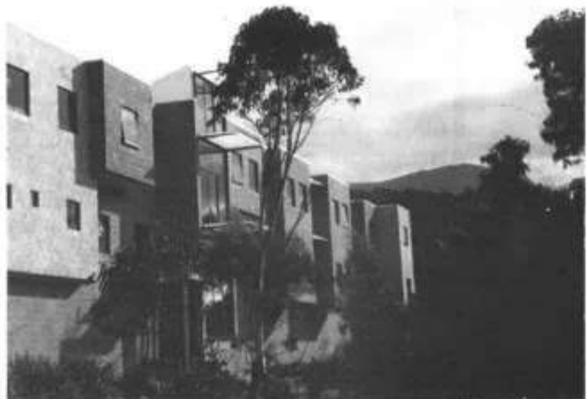
The new CSIRO/CRC building, on campus at the University of Tasmania.
