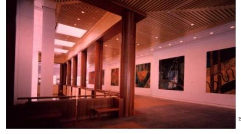
top level showing the turpentine clad columns and silver ash batten acoustic ceiling
