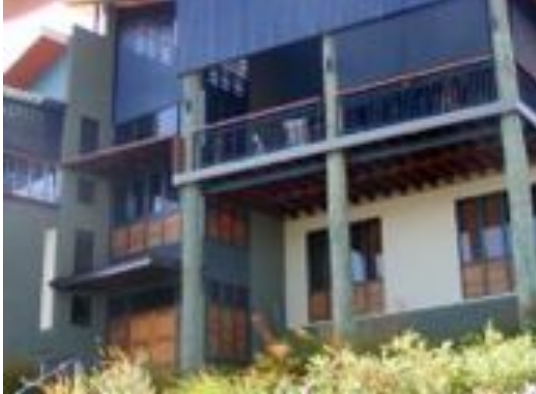
pole house, Townsville, Qld Photo: Geoff Boughton
