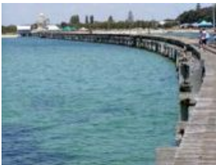
Bussleton Jetty, WA Photo: Geoff Boughton
