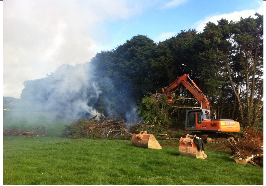
Cypress pine hedges are being removed from the milking platform
